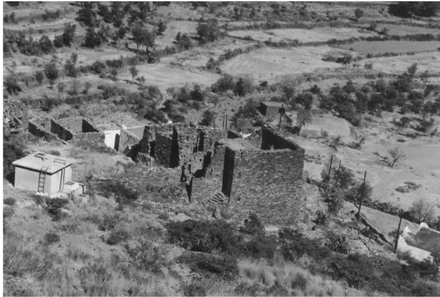
Figure 9: A deteriorated buildings in an abandoned village
