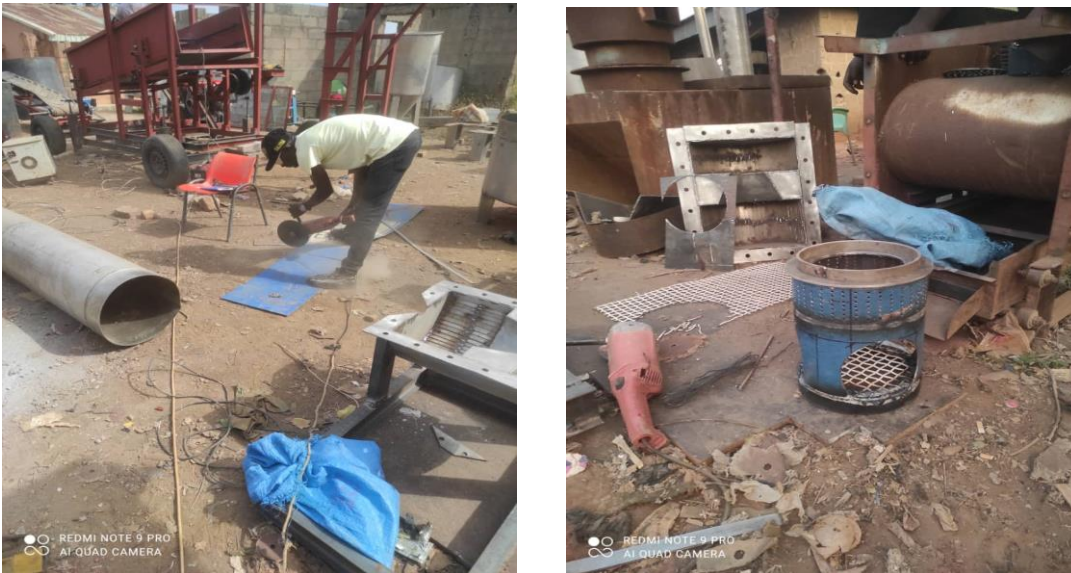
Figure14 Fabrication of dual stove components
