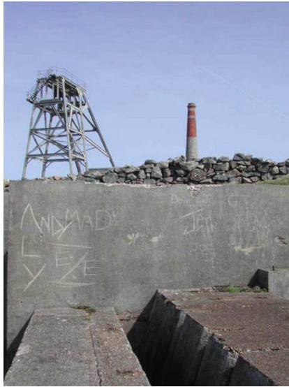
Figure 2. 20th-century remains at Botallack. The base of the Californian stamps with the headframe of Allen's Shaft in the background. Are these old enough to be considered archaeology?
