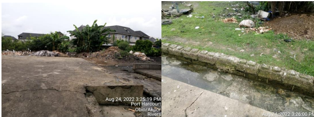
Plate II: The concreted floor and channels of waste flow
