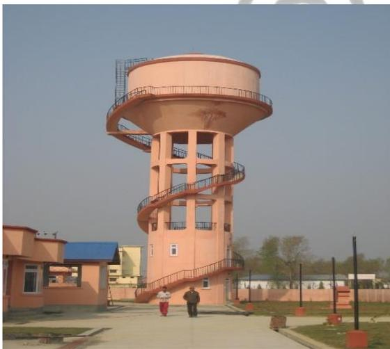
Figure 1 Elevated water tank with frame type of staging
