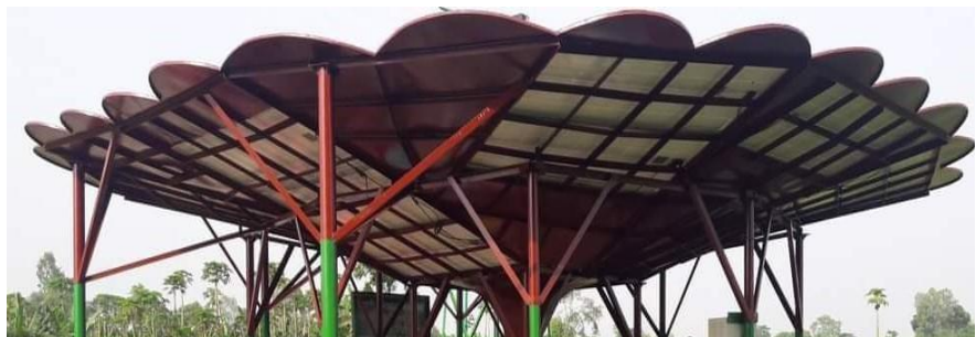
Fig. Funnel above a dug well used as a rainwater receptor.
